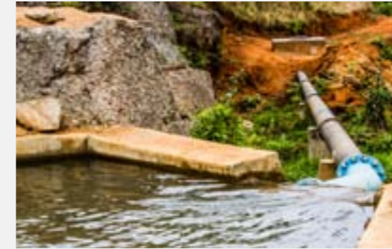
Ezulwini Water Supply
