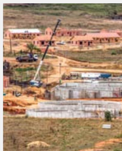
Matsapha Waste Water Treatment Plant
