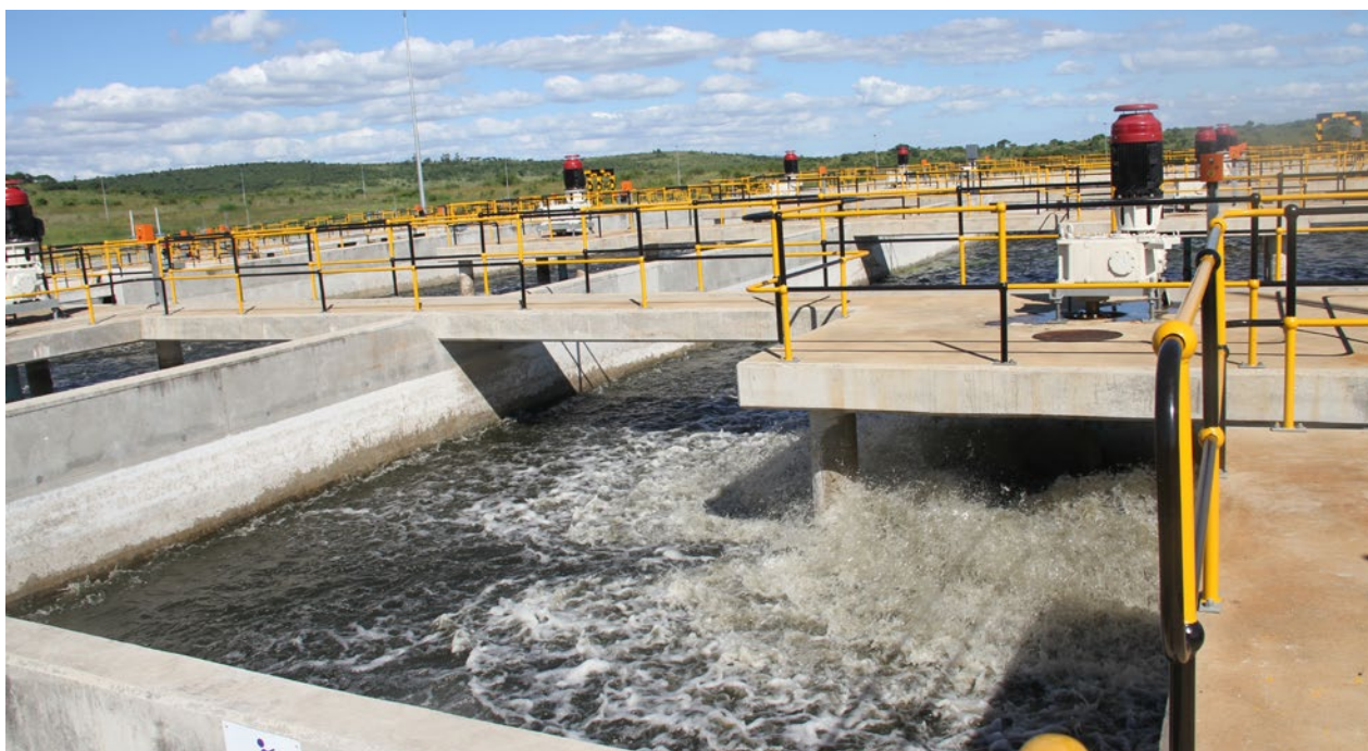
Wastewater treatment bioreactors at the Matsapha Wastewater Treatment Plant.
